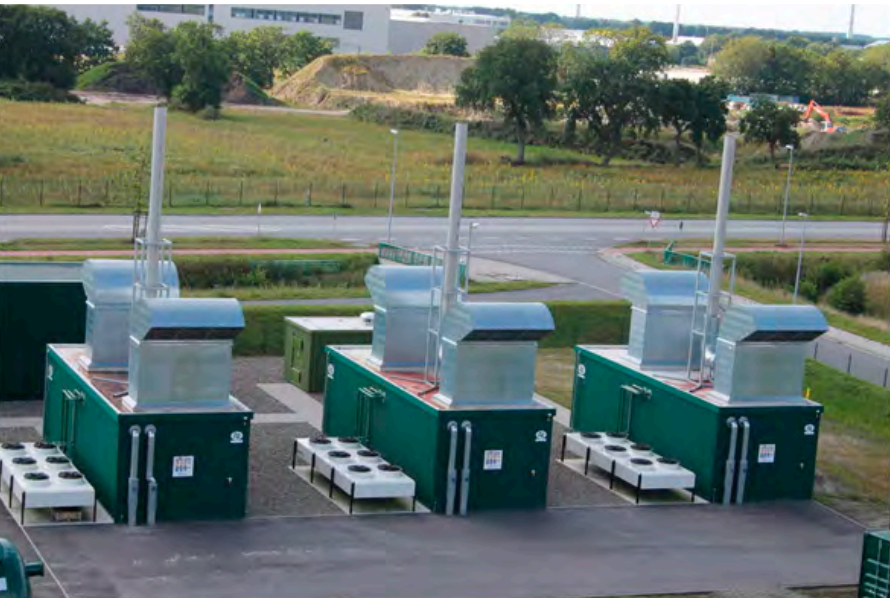
Figure A.55: CHP Generator
