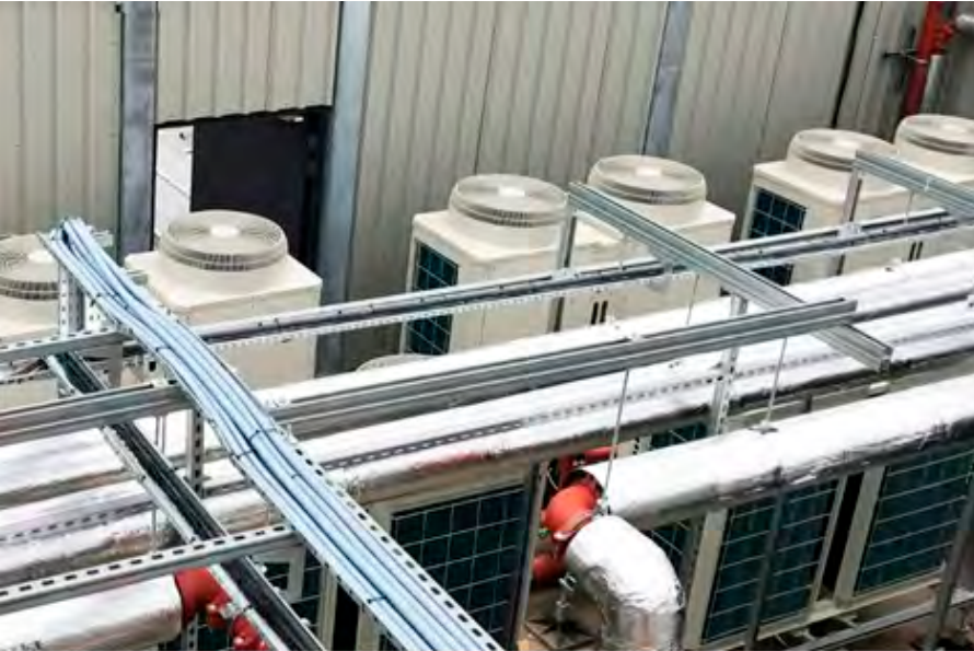
Figure A.56: Air Source Heat Pumps
